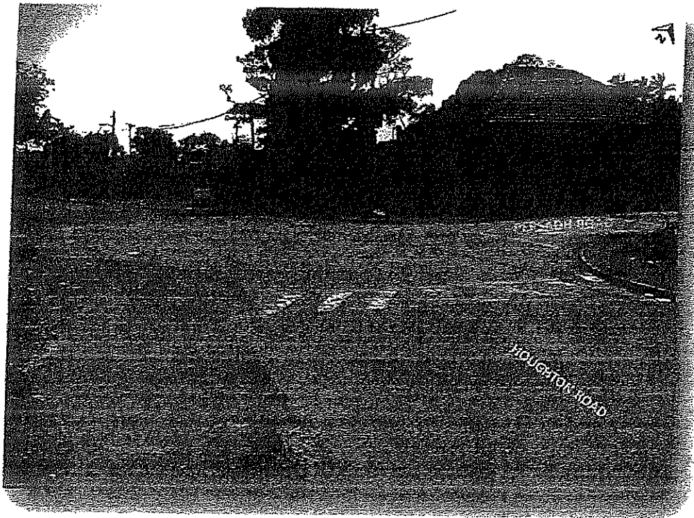
Figure 7: Intersection of Persadh Road and Houghton Road facing north west
